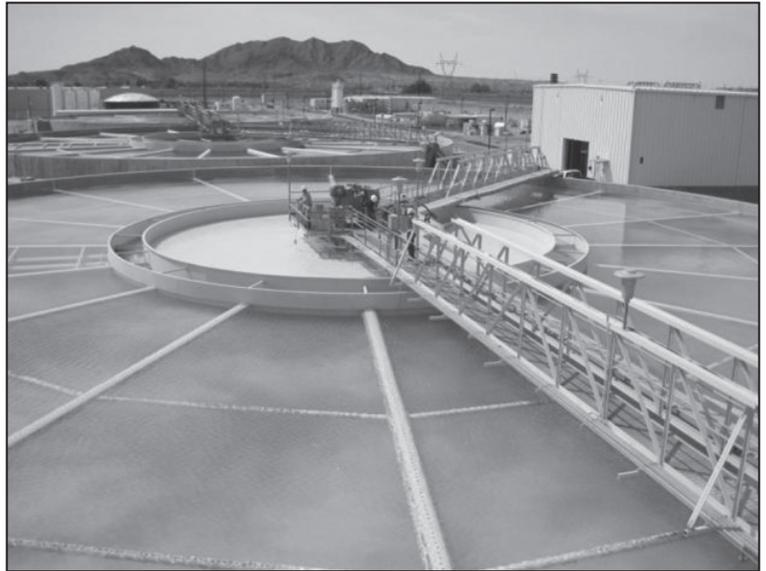
*Solids Contact Reactor in operation during Pilot Run. Photo: U.S. Bureau of Reclamation.*
