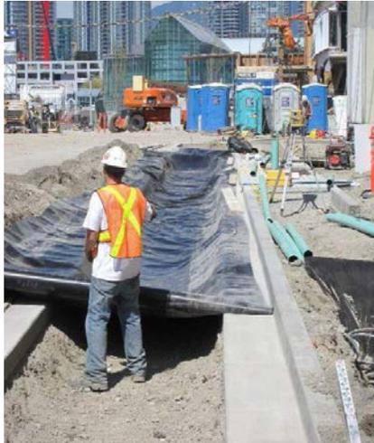
Figure 9.1. Installation of a geomembrane.
