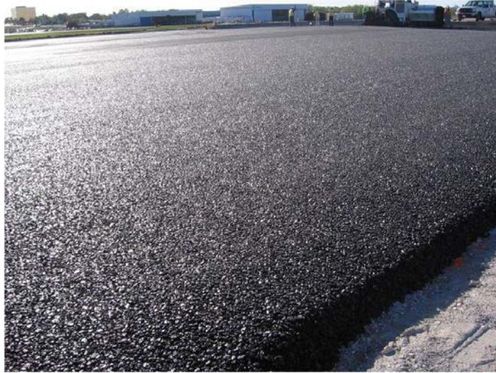
Figure 9.12. Completed porous asphalt installation.
