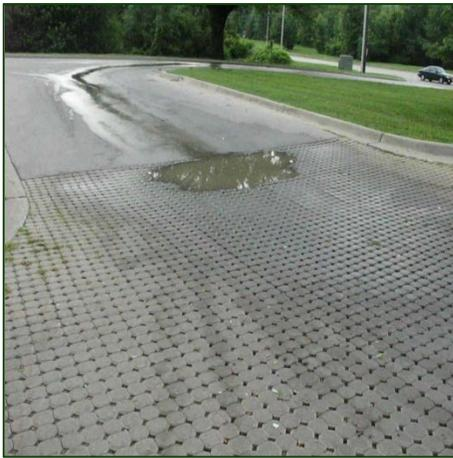
Settlement and ponding at a transition between a permeable and non-permeable pavement. The transition is poorly chosen as a low point.
