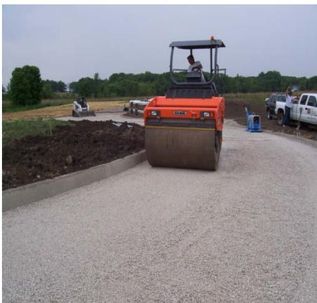
Smooth wheel steel drum compaction equipment for permeable base aggregate.
