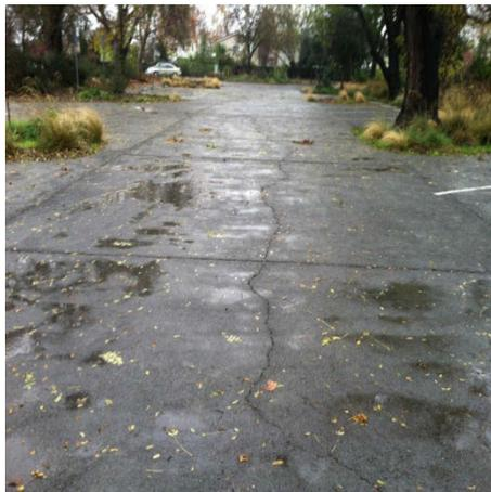
Pervious concrete parking area. Note the surface ponding, leave contaminants on the pavement and cracking of the slabs. Small aggregate was used and the resulting higher cement content may have contributed to the surface cracking.
