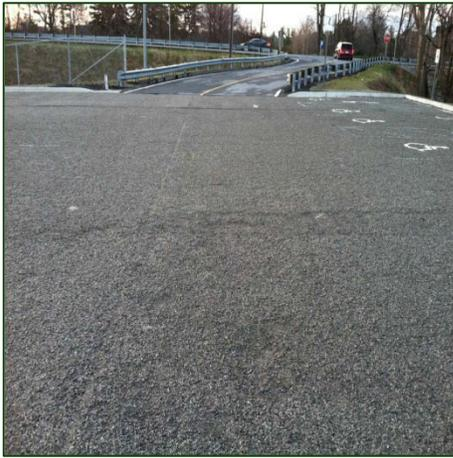
Severe raveling caused by late season concrete placement, inconsistent consolidation and inadequate curing of the concrete.
