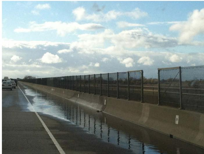
Figure 1.1. Ponding on highway shoulder.
