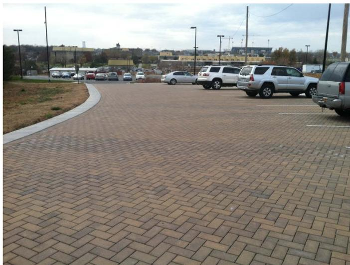
Figure 9.14. Typical permeable interlocking concrete pavement installation.
