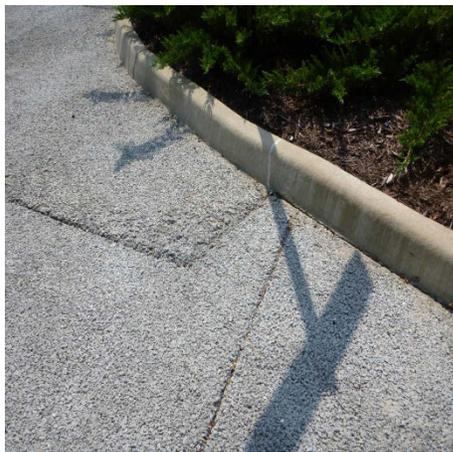
Surface raveling and poor joint treatment.
