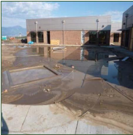
Failure to properly protect the permeable pavement during an intense storm at the time of construction.
