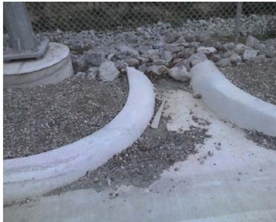
Figure 9.6. Example of a curb cut-out.
