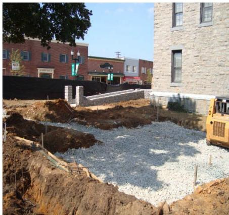
Stone reservoir aggregate should be protected from contamination from the surrounding area by grading the area away from the stone reservoir or using protection devices such as silt fences. (Photograph shows poor protection).
