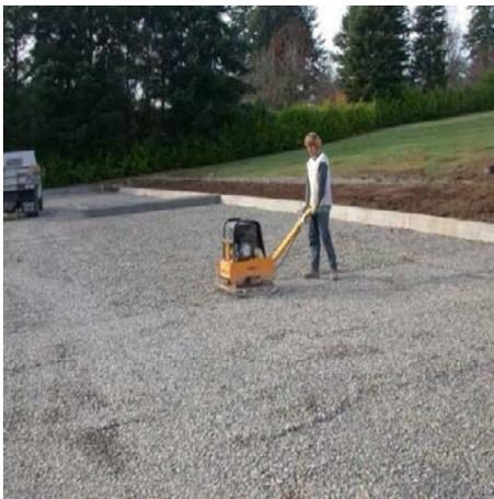
Compaction should be completed using appropriate equipment for the area and thickness of the aggregate layers. The equipment shown would likely result in non-uniform compaction.
