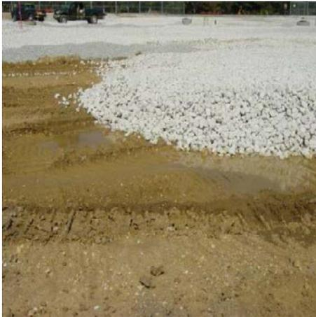
Contamination of the subgrade should be avoided by end dumping the stone reservoir aggregate and spreading it forward using a bulldozer.
