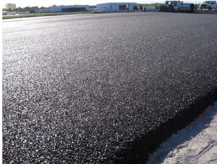
Figure 3.3. Porous asphalt pavement.
