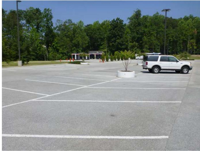
Figure 3.4. Pervious concrete pavement.
