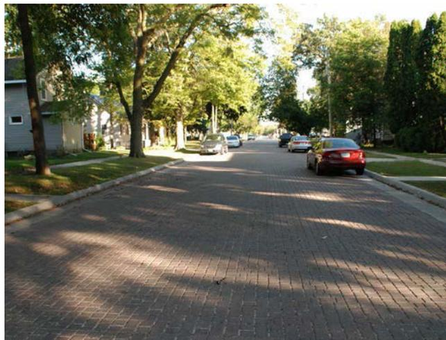
Figure 3.5. Permeable interlocking concrete pavement.
