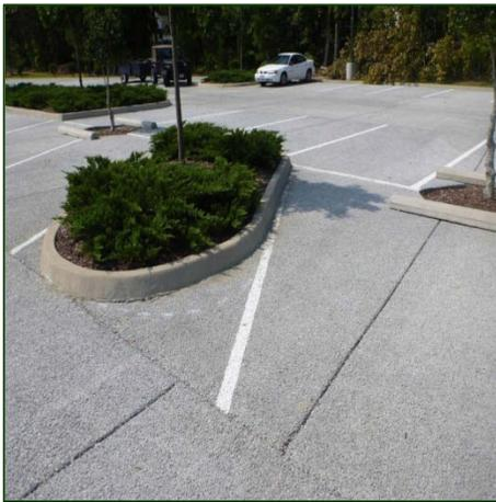
Minor joint raveling. Poor selection of joint locations leading to cracking of the pervious concrete.
