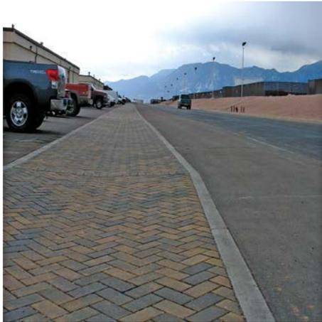
Permeable strip paving to improve localized drainage issues. Note the concrete curb adjacent to the asphalt paving to the right.
