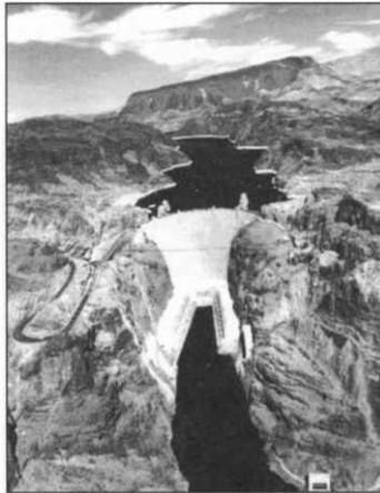
*The energy/water nexus writ large. The decline in Lake Mead's elevation since 1999 prompted the Bureau of Reclamation to initiate a program to modify the turbines at Hoover Dam to increase their electrical generating capacity at lower lake levels.*
