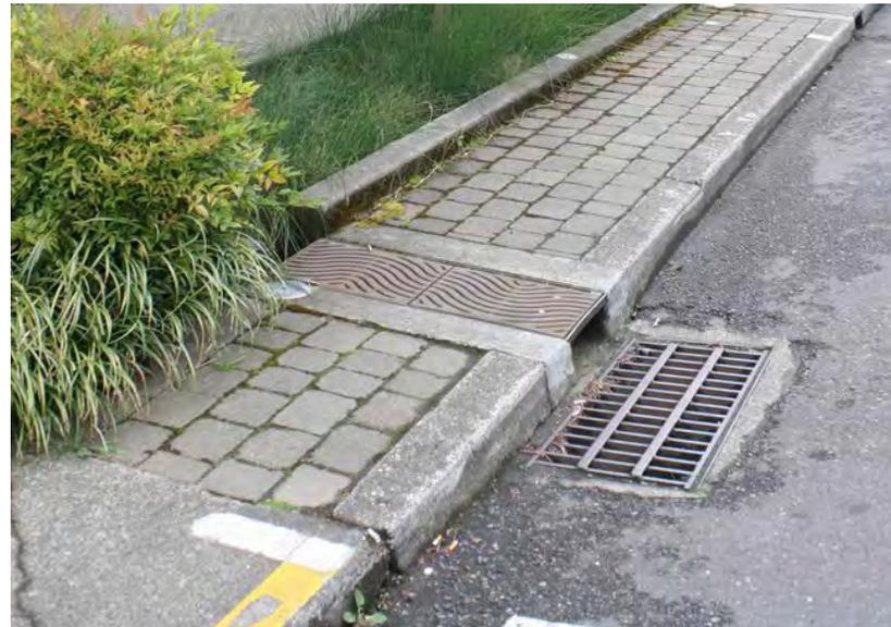
A Grated Curb Cuts conveys stormwater across a sidewalk
