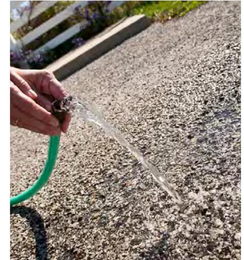
Porous asphalt paving is a runoff-reducing in paving areas and driveways.
