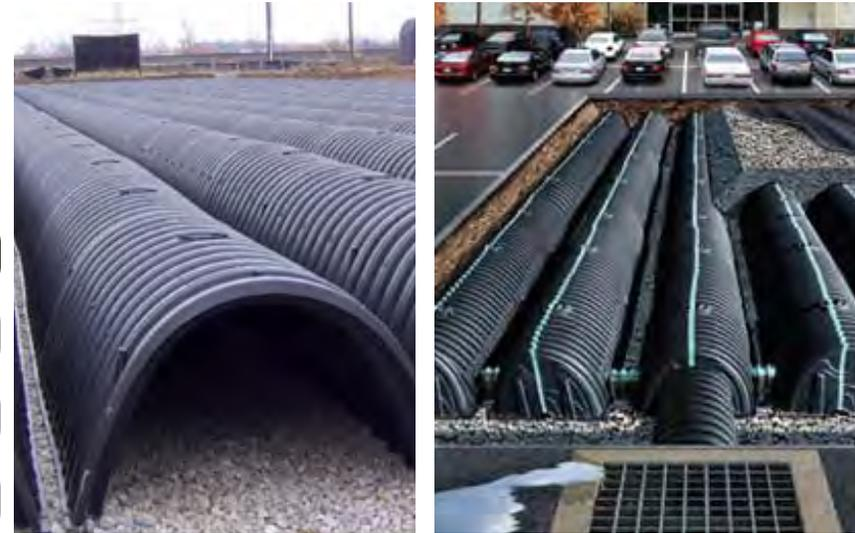
Drainfields provide for a large volume of stormwater storage and promote groundwater recharge.
