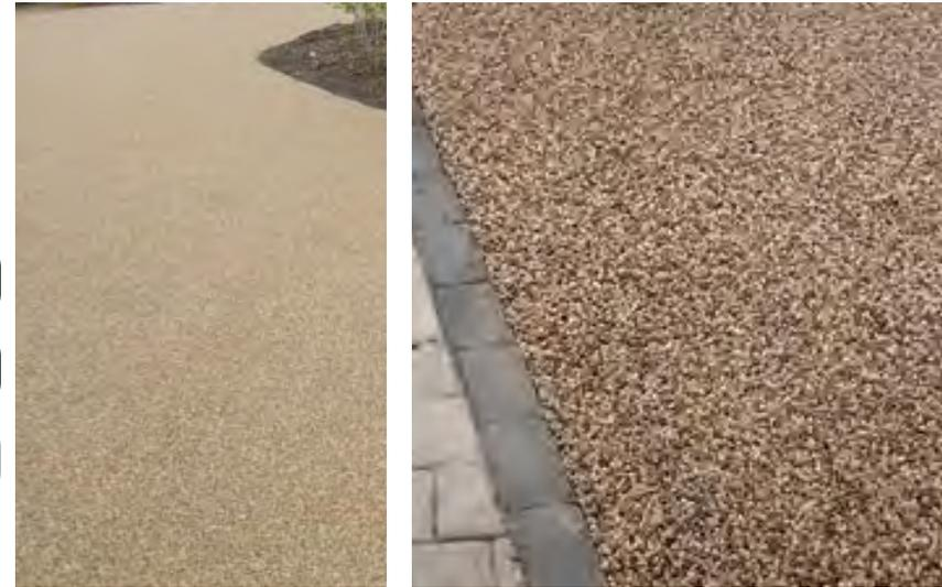
Stabilized aggregate reduces storm runoff from low-traffic paving areas.
