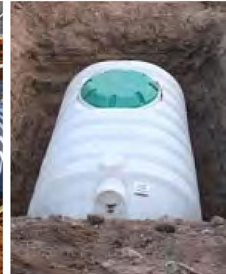
Underground cisterns provide storage areas for rainwater reuse.
