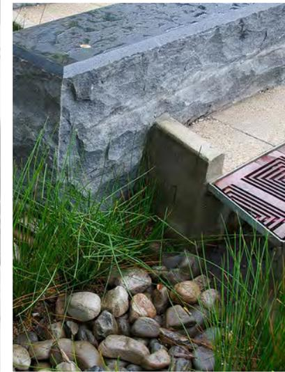
Bioretention cells fit into constrained urban site.
