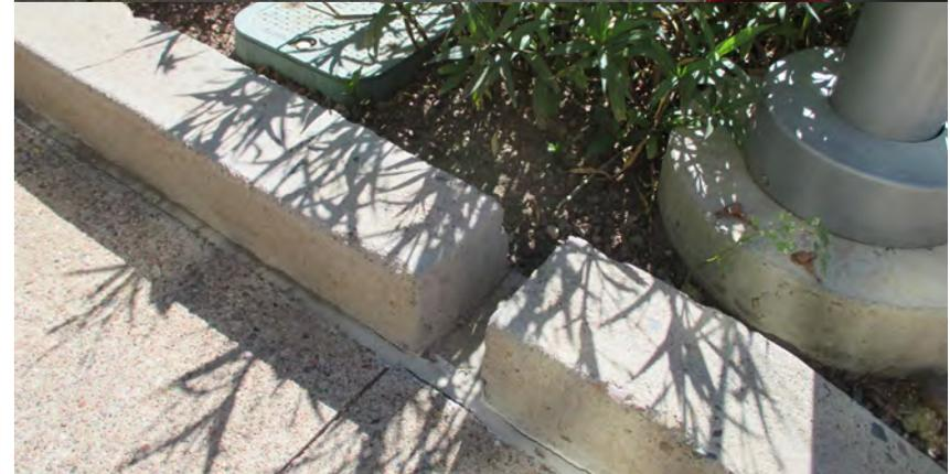
Standard curb cuts open up planting areas to receive stormwater flow.
