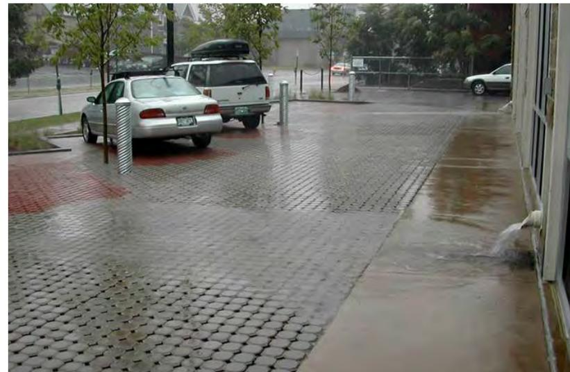
Permeable Pavement can capture most stormwater runoff.
