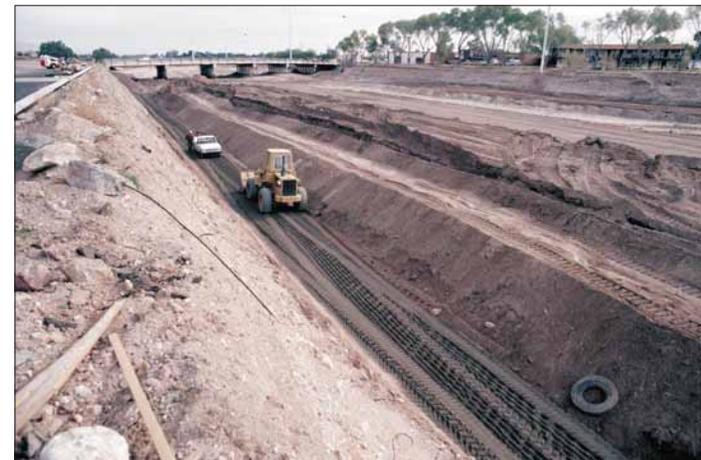
*Figure 4-4 Bank stabilization structure under construction west of Campbell Avenue.*
