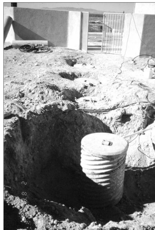
*Figure 3-14 Cistern installed as part of a graywater reuse system. Photo: Val Little.*
