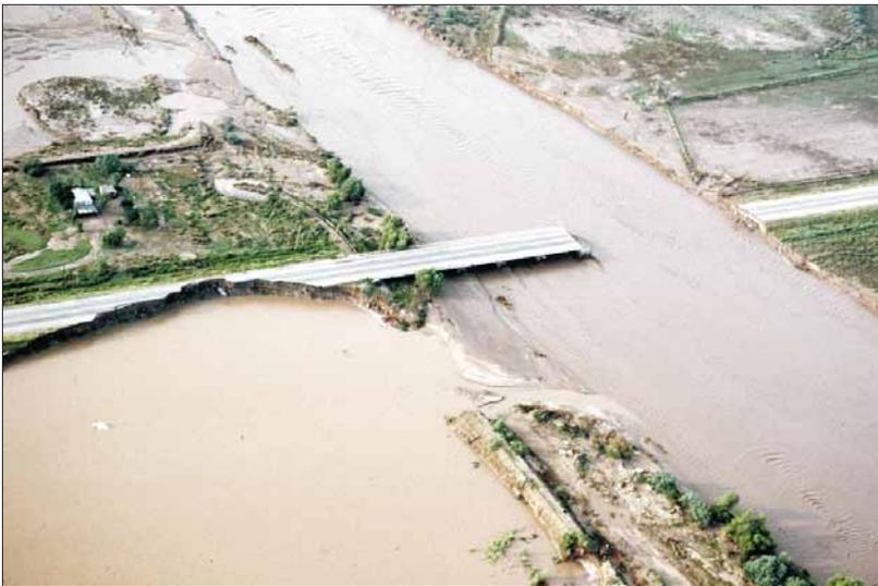
*Figure 4-6 Floods damage the Ina Road Bridge.
