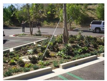
Figure 3. Parking lot runoff captured by bioretention in parking islands
