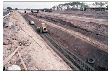
Figure 4-4 Bank stabilization structure under construction west of Campbell Avenue. Photo: Peter Kresan.©
