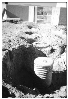
Figure 3-14 Cistern installed as part of a graywater reuse system. Photo: Val Little.
