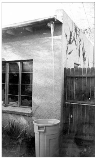
Figure 3-15 A do-it-yourself water harvesting system collects rain from roof for use to irrigate a home garden. Photo: Barbara Tellman.
