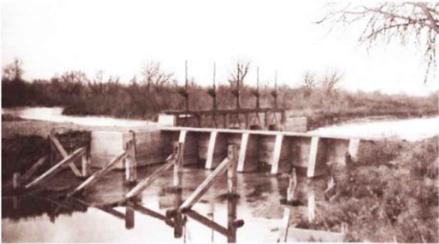
(1925): Diversion Point. Canal has been in place and diverting water for 120 years.
