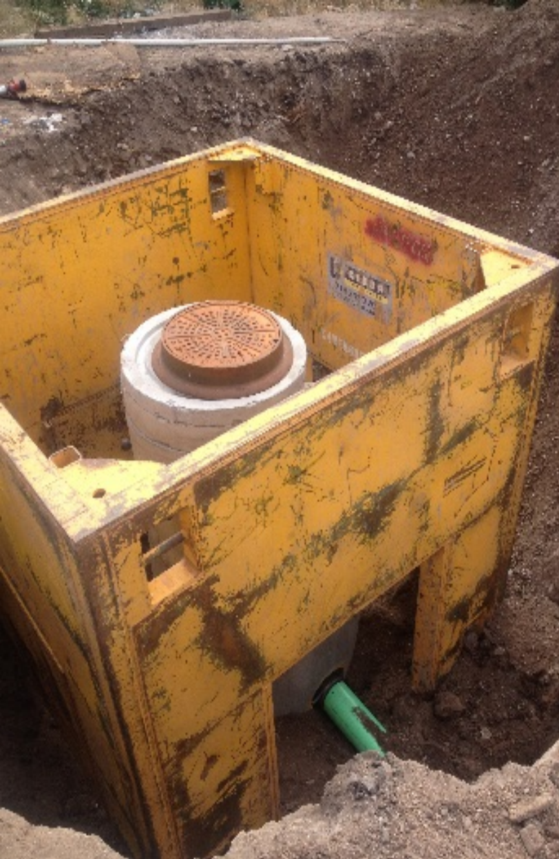
Manhole Construction
