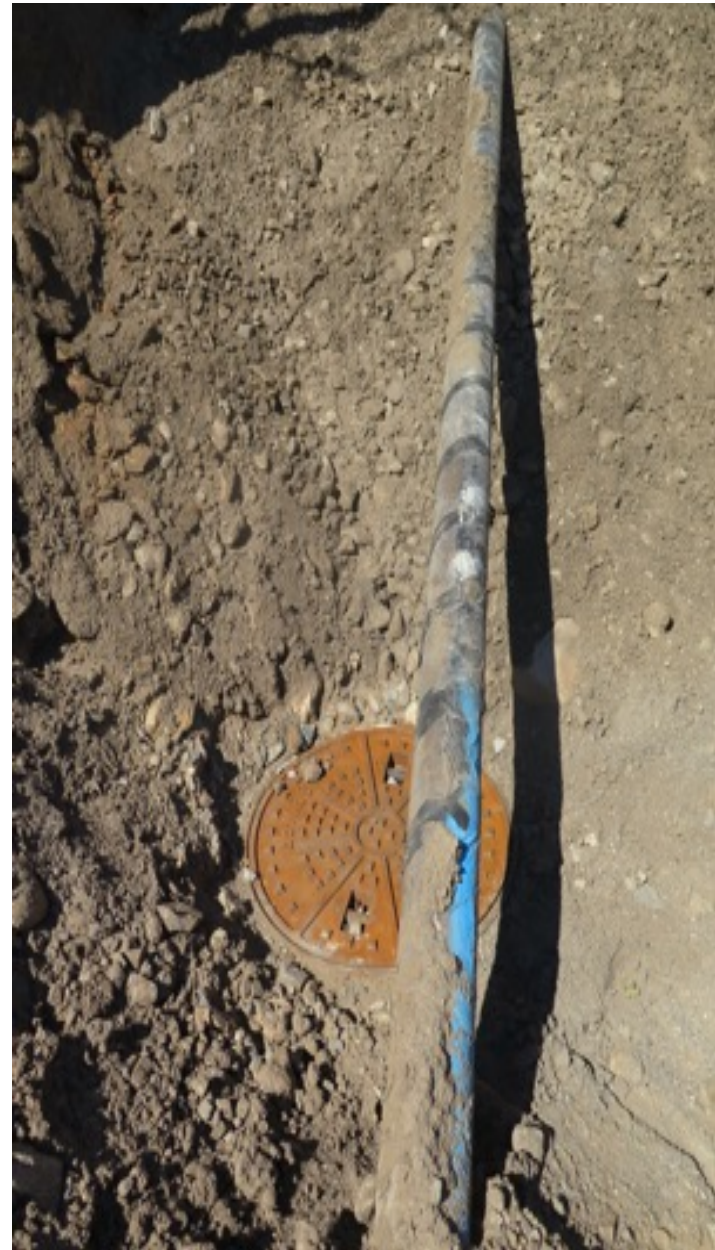
Waterline Above Sewer Manhole (Waterline Will Be Moved)
