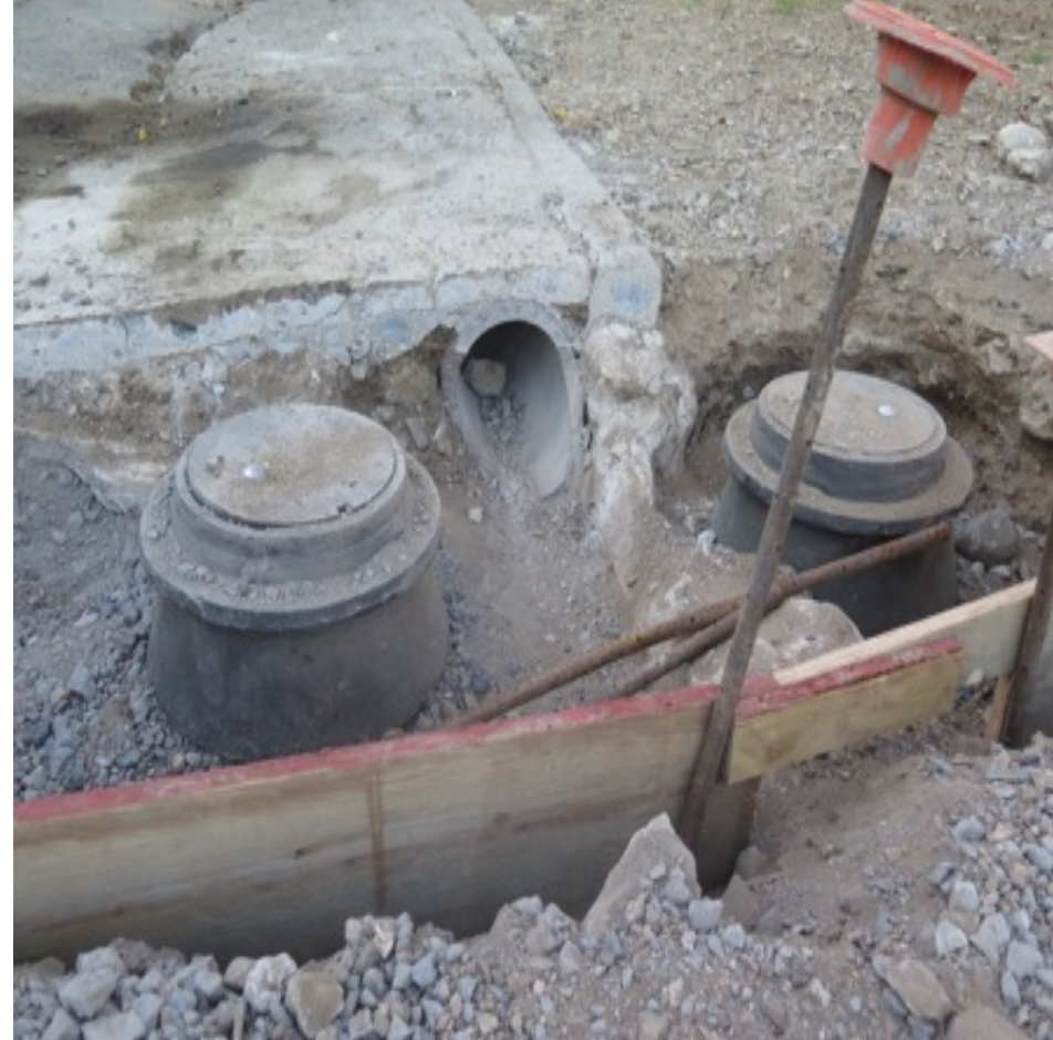
Cleanout and Backwater Valve Installation
