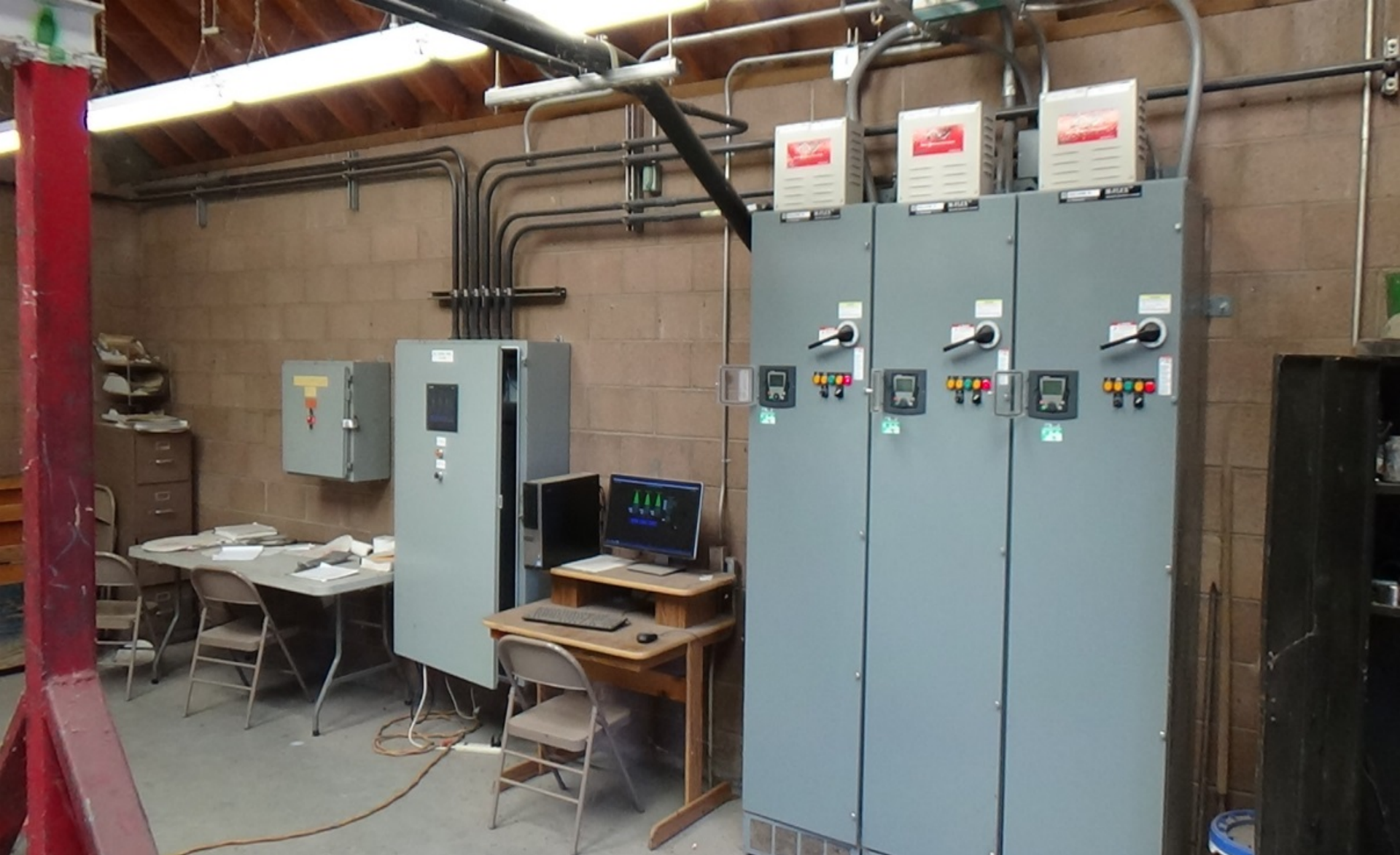
Pump and Variable Frequency Drive Control Panels, SCADA System
