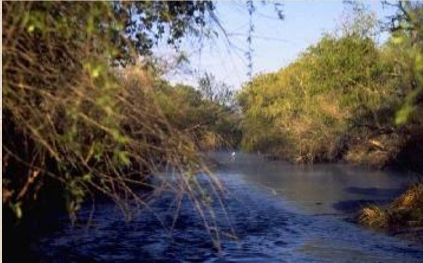
91 st WWTP Outfall into Salt River
