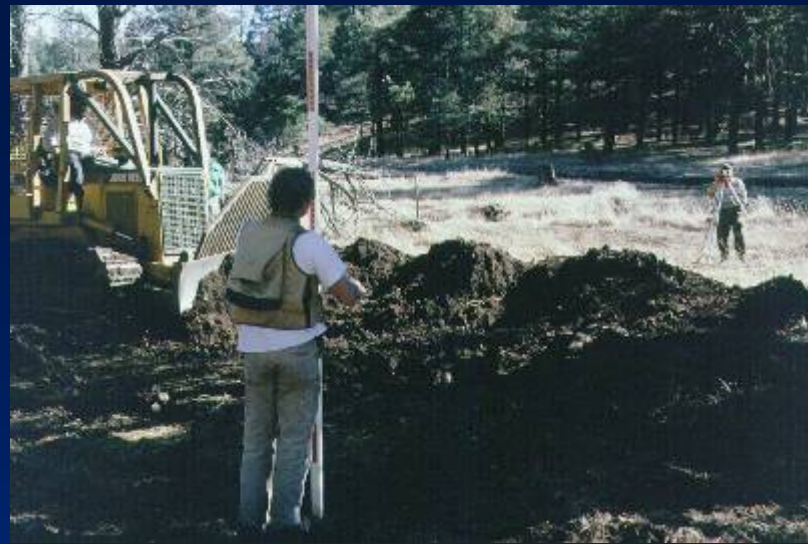
Earth moving, November 1998
