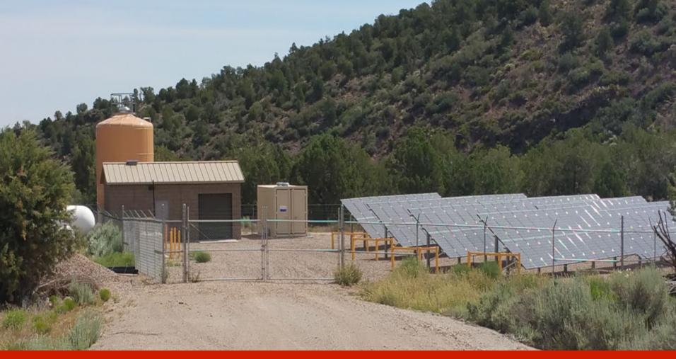
Westwater Well, recently upgraded to combine water from two wells and deliver Water to Grand Canyon West, through a new upgraded 6" water line. Concerns are that the aquifer is a perched aquifer and we monitor quantity to ensure that not too much water is pumped from the wells to ensure that we maintain a positive recharge capability
