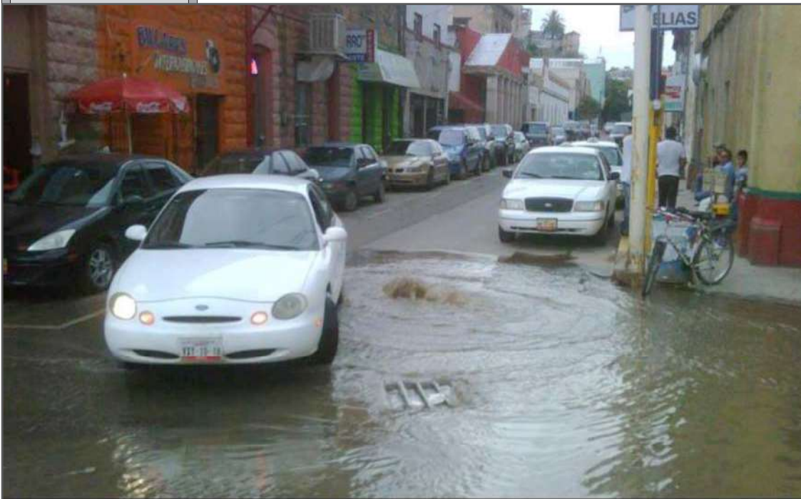
Figure 1: Wastewater overflow in Nogales, Mexico. Photo courtesy of Hans Huth.
