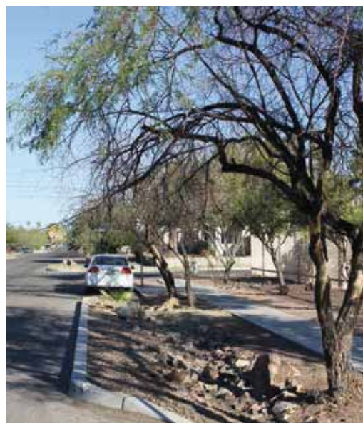
Left: Rincon Heights bump-outs harvest stormwater and protect pedestrians and parked cars. Photo by Sandra Bolduc, PCRFC
