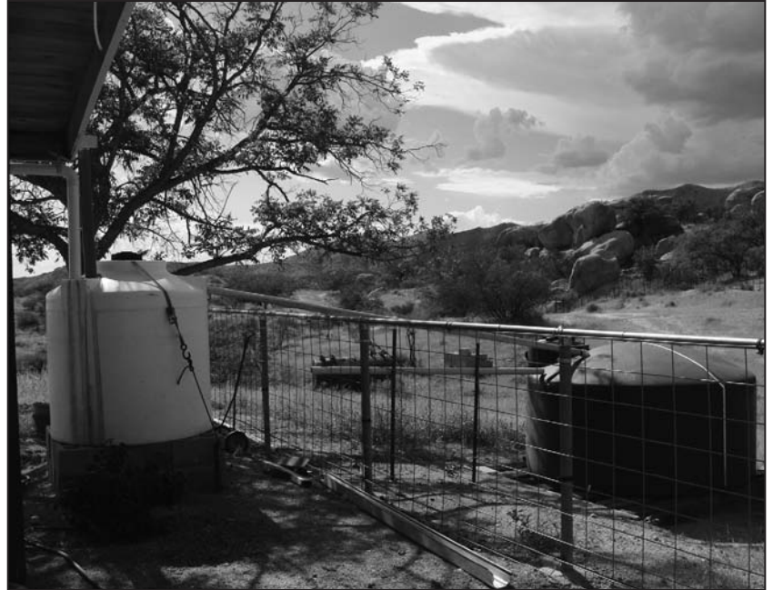
Water harvesting tank collects rain water from the roof at the 4Y homestead.
